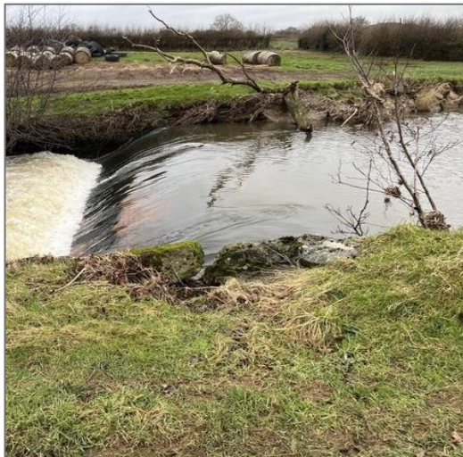
A weir on the River Otter below Honiton. This acts as a partial barrier to fish migration. Historic straightening of the river channel and cattle grazing of the river bank has led to increased erosion and poor habitat
